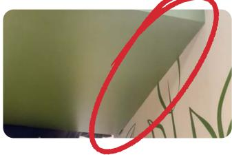
When fitted correctly, the top arch panel will be flush with the end panel.
