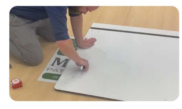
Step 5 Turn the panel over, and go through the cuts at the back of the panel with the Stanley Knife.
